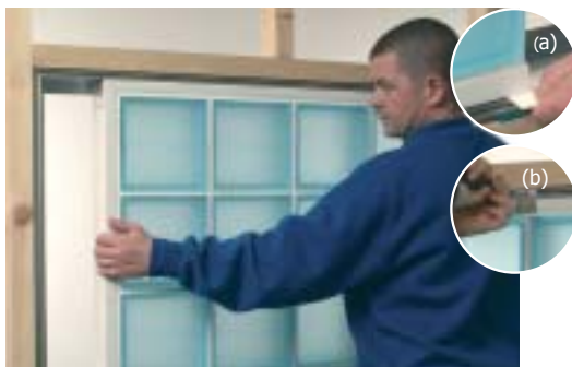
Step 2 : Vertically lift the first panel having placed plastic packers on base of aluminium (a) and slide into position. Temporarily secure in place using restraint anchors (b) supplied.
