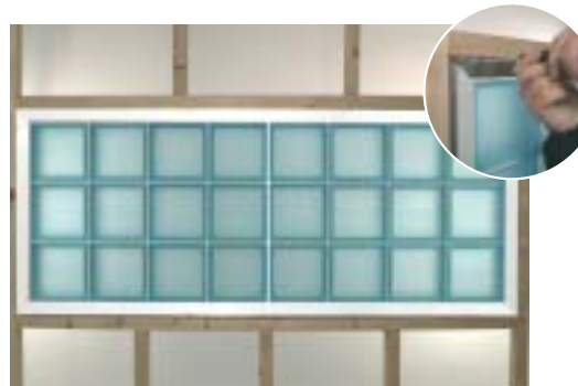
Step 4 : Position second piece of channel and screw bolts into pre-drilled holes. Note : Fit sides first, then top, then bottom. If the Precast Easifix is a vertically or horizontally connecting panel, grout the connecting joint, both sides with the grout supplied.
