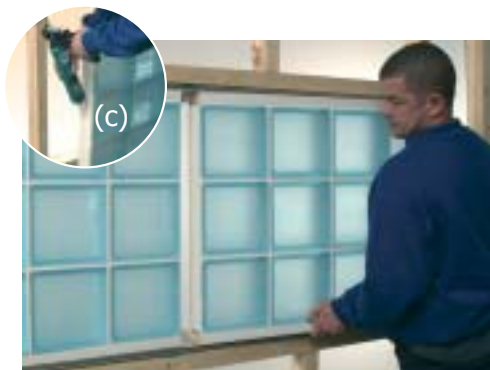
Step 3 : Apply silicone to the connecting joint on the second panel (c). Carefully lift second panel in vertical motion onto plastic packers and slide up to first panel ensuring a neat joint at intersecting point. Note : Apply more silicone if required.
