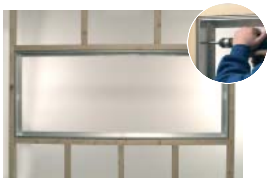
Step 1 : Position and screw in place first part of aluminium channel. Ensure that the screws are located to the relevant marker.
